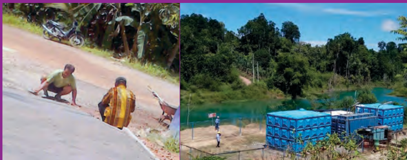
Concreting of village road
