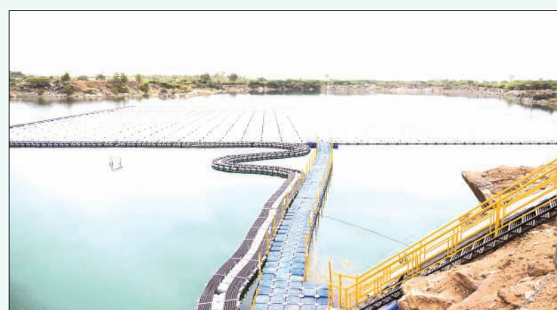
Floating Solar Plant at UCWL
