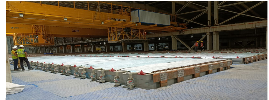
Refinery Cells commissioned
