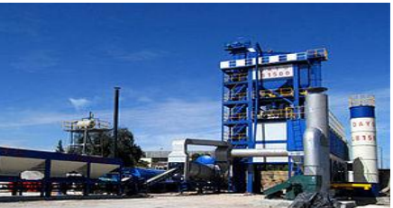
Contractor Camp Mobilization
