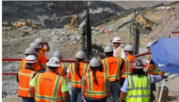
Construction at site
