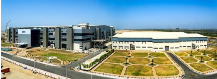
State of art facility of 1.5 GW premium Solar cell and modules manufacturing facility located in India's largest electronic manufacturing cluster
