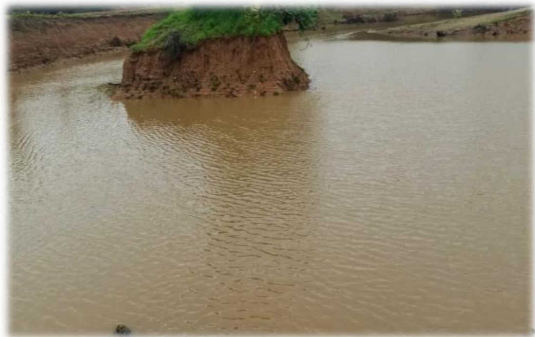
Pond renovation for water harvesting and ground water recharge
