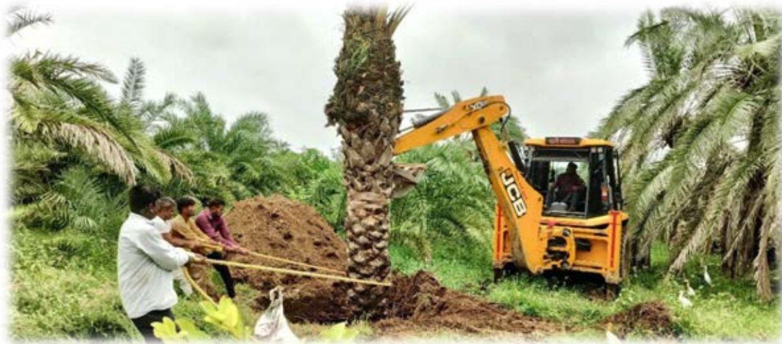
Photo: Date restoration activities.
